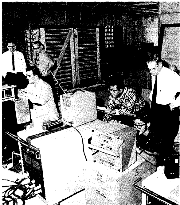
Staff and students conduct vibration tests of Millikan Library
