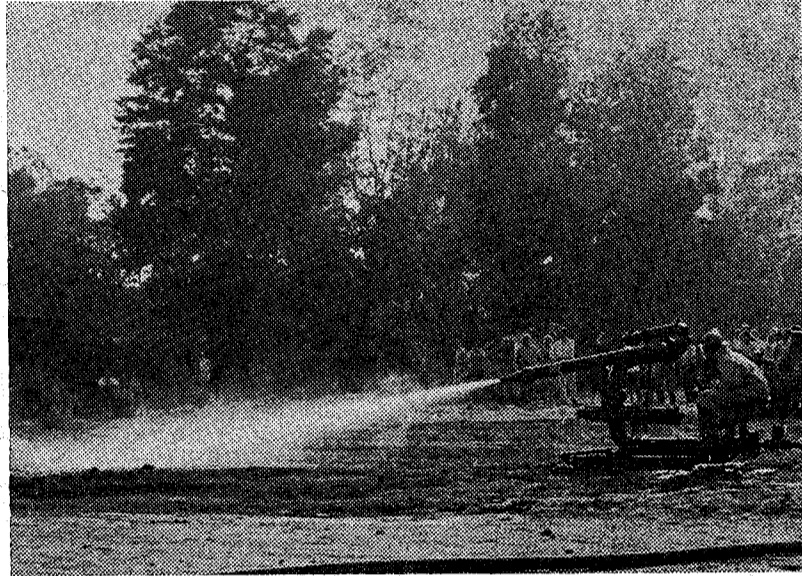
A placer mining gun breaks ground for the $2.5 million Keck Engineering Laboratory. The gun symbolizes the hydraulics research that will go on in the lab.
