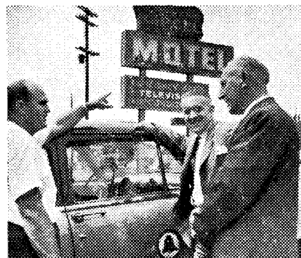
"1:30 p.m. After lunch, I look in on a PBX and room-phone installation at an out-of-town motel. The installation supervisor, foreman and I discuss plans for running cable in from the highway."
