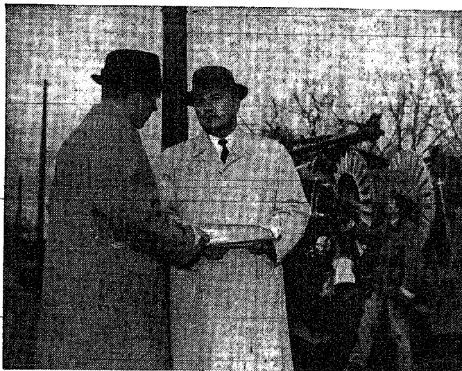
Ken Boekeloo (center foreground) at the scene of a cable installation project in Detroit.
