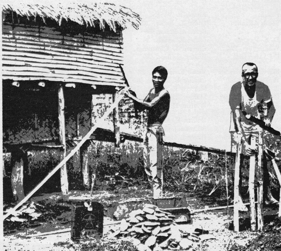
Philippines: Jim Eder helps a local resident install a drainage system for his kitchen.
