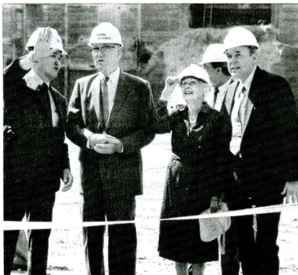
Dr. and Mrs. Arnold O. Beckman (center) with Don K. Toy and President Thomas E. Everhart at the first pouring of concrete for the foundation of the Beckman Institute. Toy is with the architectural firm of Albert C. Martin & Associates.
