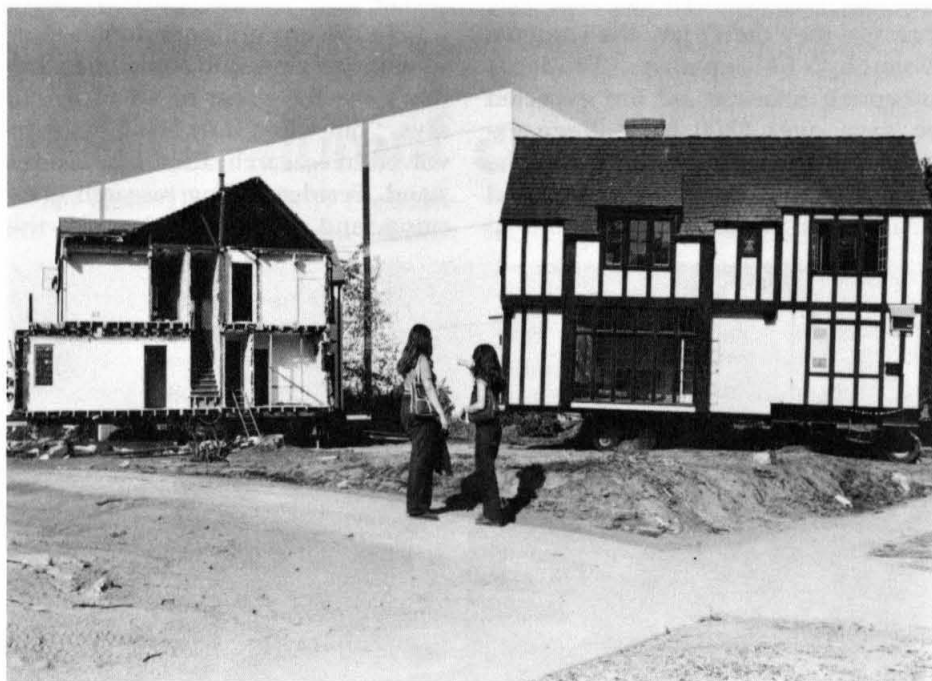
Ready to be rolled away to 1144 Lura Street where they will be united, are these portions of the former public relations house. Moved from the site of the Braun Laboratories, the house will be used in its new location for offices of the Environmental Quality Laboratory.
