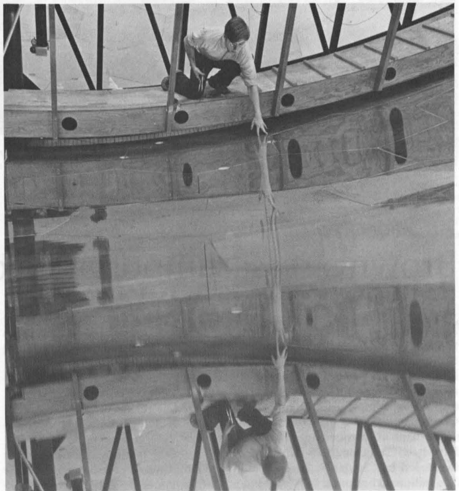
The polished surface of Caltech's new 34-foot radio telescope mirror creates surrealistic images of the hand and arm of Michael L. Norman, BS '75. The dish is to be installed at the Owens Valley Radio Observatory where it will be used primarily for studying the distribution of molecules in interstellar dust clouds.
