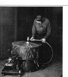
STRAND model M6 flexible shaft machine shown in this picture is used in the Optical machine shop for grinding welds, polishing, buffing, sanding, rotary filing, nut setting, and die sinking. Strand machines are built in sizes 1/8 to 3 hp—speeds 80 to 10500 R.P.M.
