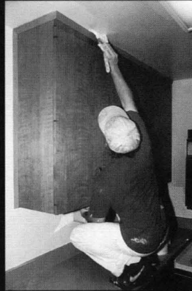
Patrick Spradlin renovating Ricketts.
