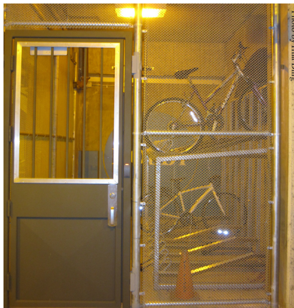
Two bikes are safely locked at night in the bike cage on the second floor of Holliston Parking structure.
