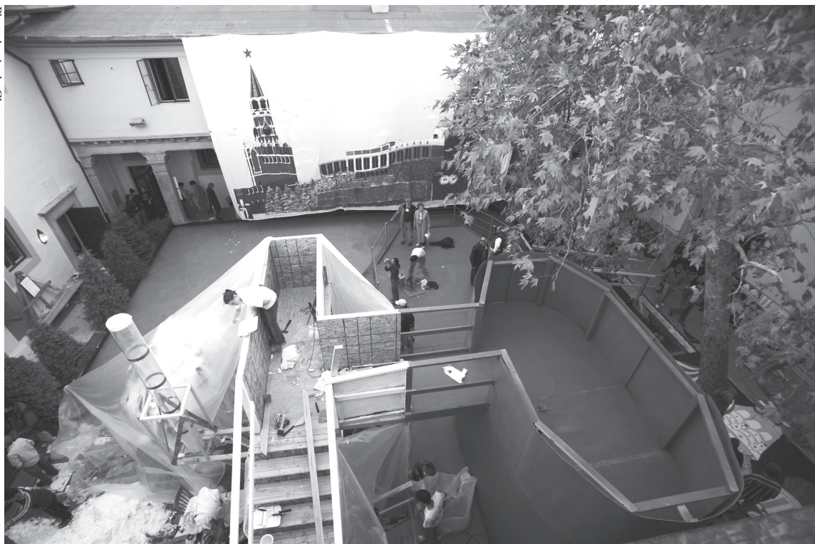
A view of the submarine in the middle of Blacker's courtyard
