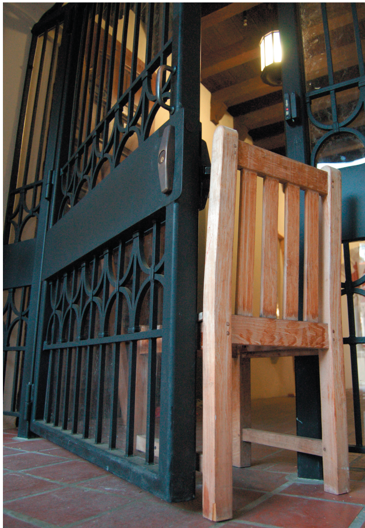
The locking mechanism of this gate, a newly installed entrance to Ricketts and Blacker hoveses, was disabled on Jan. 2
