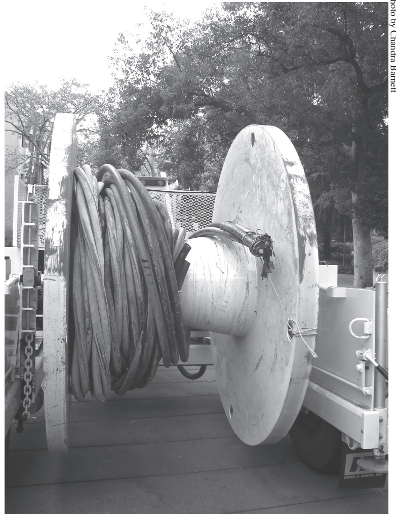
The damaged cable extracted by PWP employees
