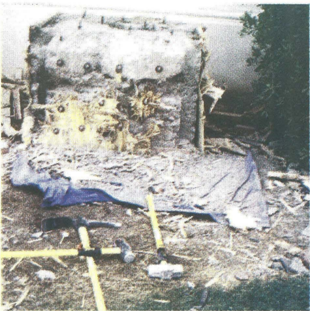
R. Forster/The California Tech "He said they'd be done a couple hours ago!" Members of Ricketts' Twilight stack take a break from their brute-force efforts to extract a key from a concrete block.
