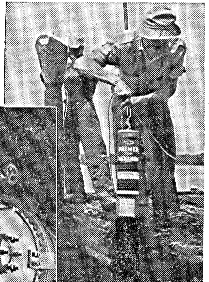
A. L. St. Peter, Princeton '37, supervisor blasting operation Susquehanna River Project, lowers a 5 1/2 inch "Nitramon" Primer into one of 600 drill holes preparatory to blasting a pipe line ditch.
