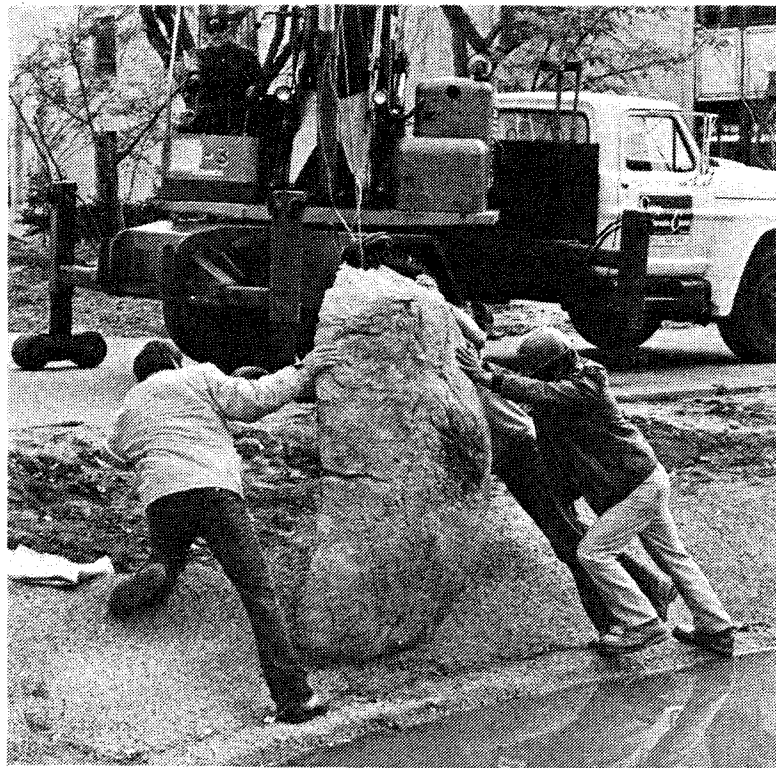
THROOP SITE GETS ITS ROCKS ON as part of current landscaping designed to disguise the area as a verdant paradise. Photo by Feeney
